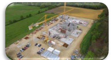
Construction Tréauray II
